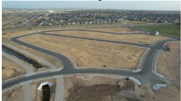
Western Half of Site (Looking Southwest)
