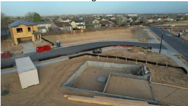
Proposed Pond – Along East Side of Site (Looking Southeast)
