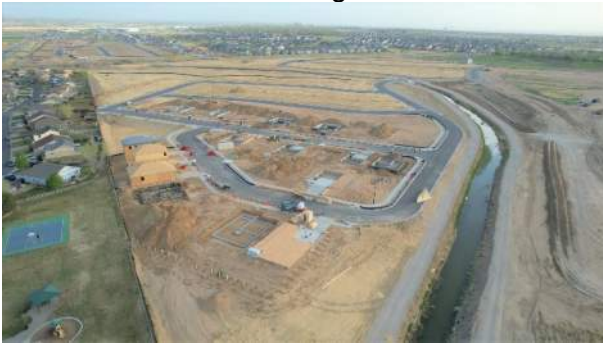
Aerial facing South
