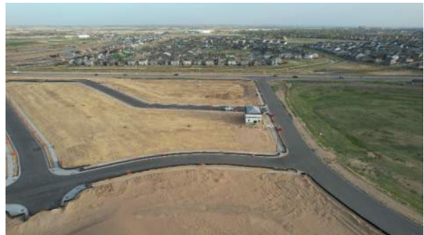
Proposed Pond - Southwestern corner of Site (Looking South)
