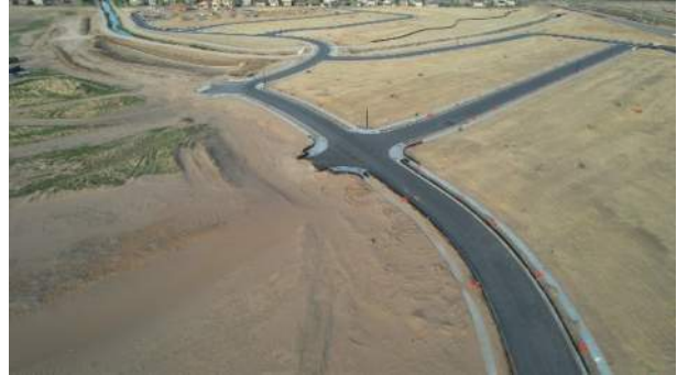
Pinnacle Avenue (Looking East)
