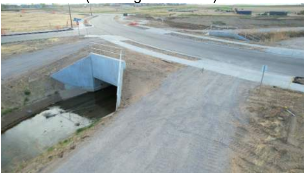
Slurry Wall at Ledge Street Crossing Over Speer Canal
