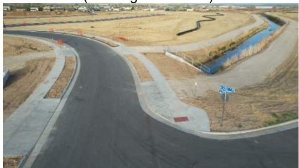
Ledge Street Crossing Over Speer Canal (Looking East)
