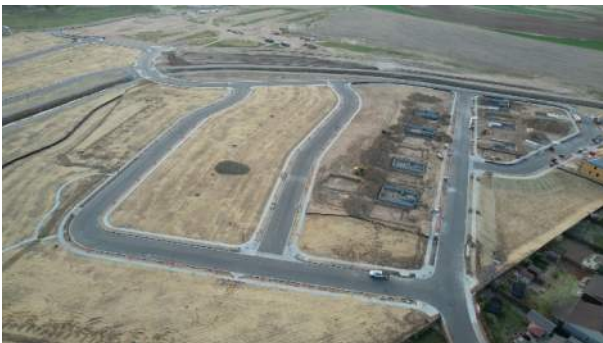
Eastern Half of Site (Amendment No. 3) (Looking Northwest)
