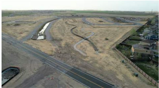
Aerial facing West
